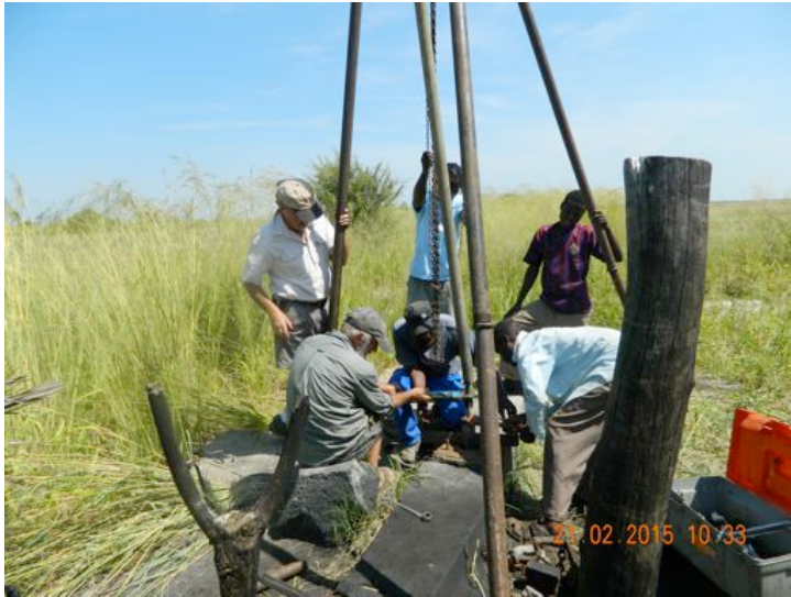
Pulling the borehole pump out at Corner Pan
