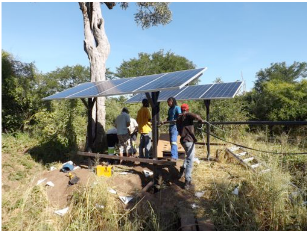
Installing the pump at Inyantue Dam borehole
