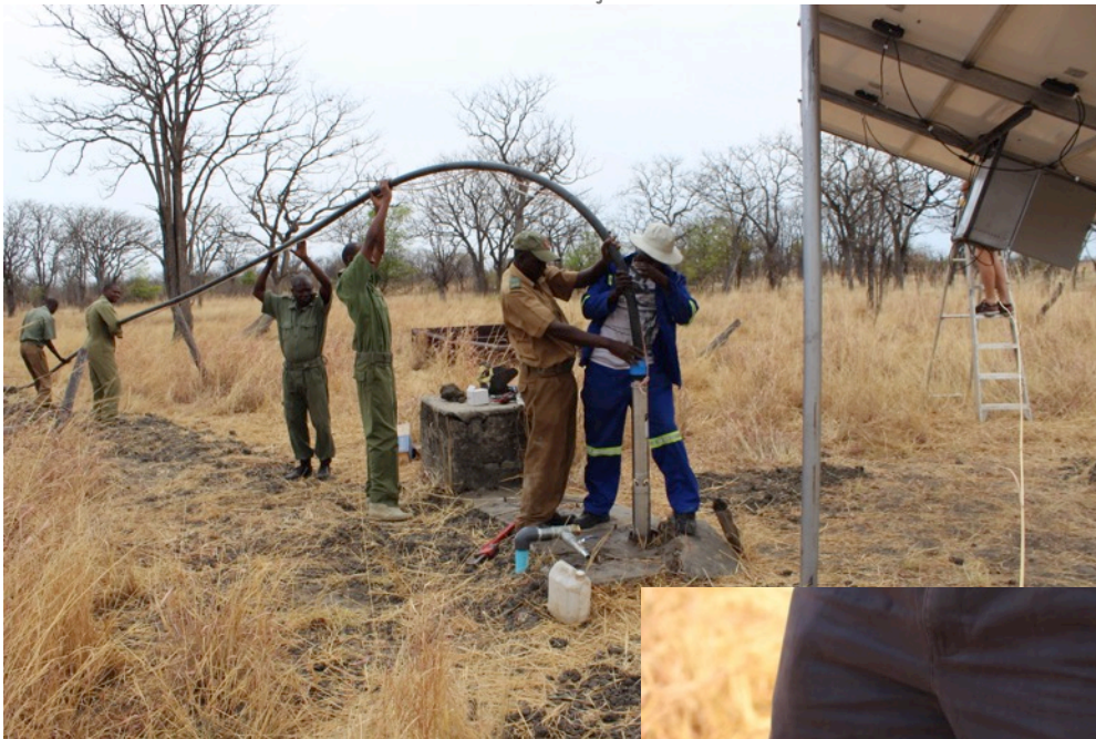
Top – putting the pump in at Roan Pan
