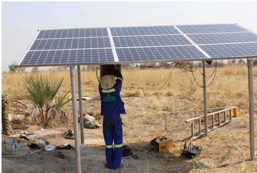
Kazuma Pan – wiring up the solar panels
