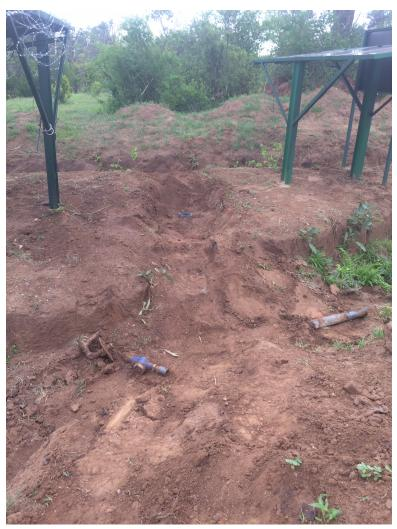
The pump at Timots Pan was totally trashed by elephants! They managed to push in part of the trench to cross over and pulled off the pipeline connection, the meter and the pump head, leaving just the top of the borehole pipe exposed. The pump restraining rope snapped and the pump dropped down the borehole. However, we have retrieved it and in early January will reconnect the whole system, plus put in better protection.
