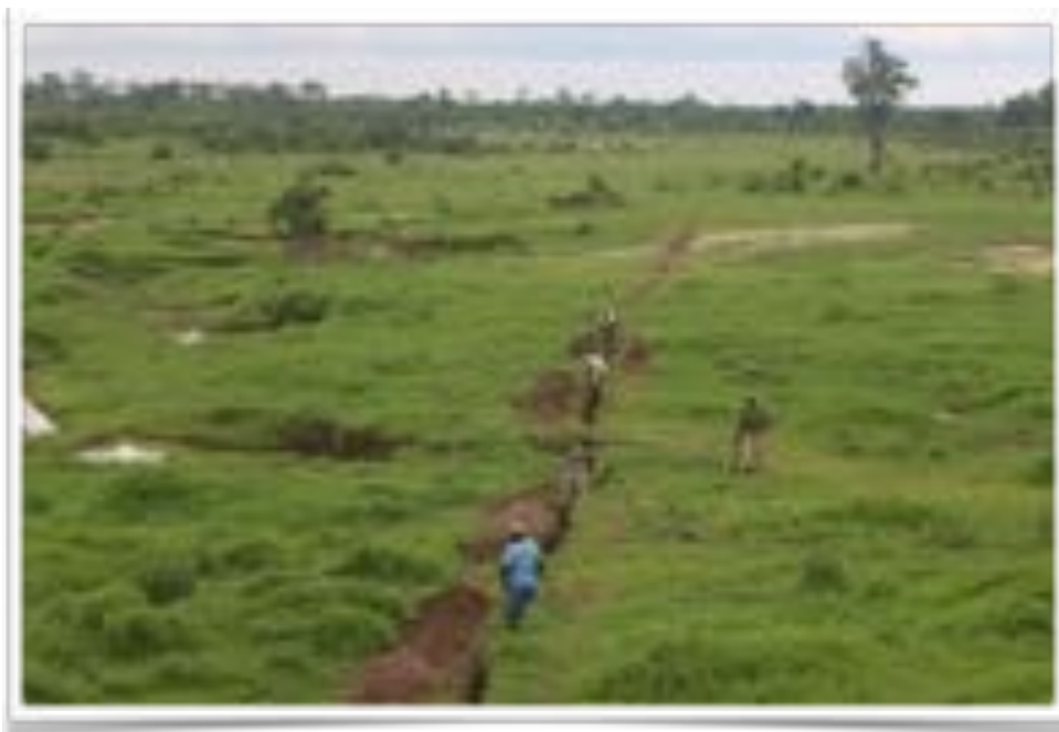
Digging the new pipeline at Deteema Dam
